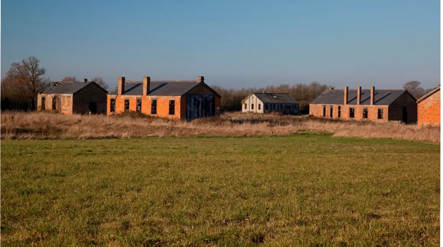
Buildings at Stow Maries
