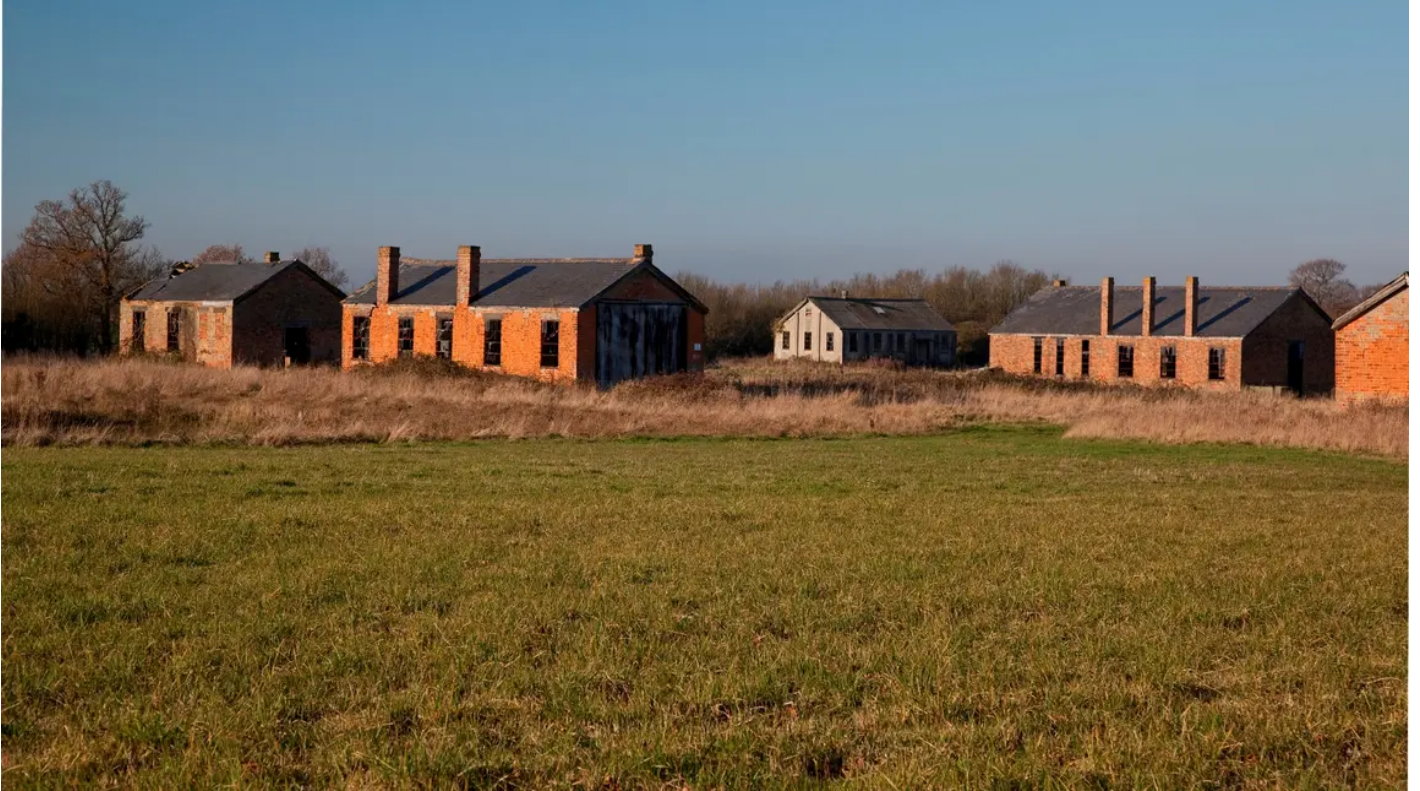
Buildings at Stow Maries
