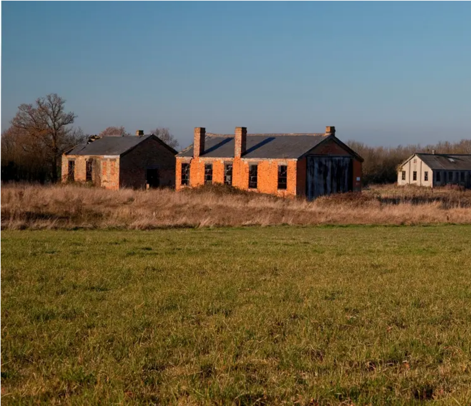
Buildings at Stow Maries
