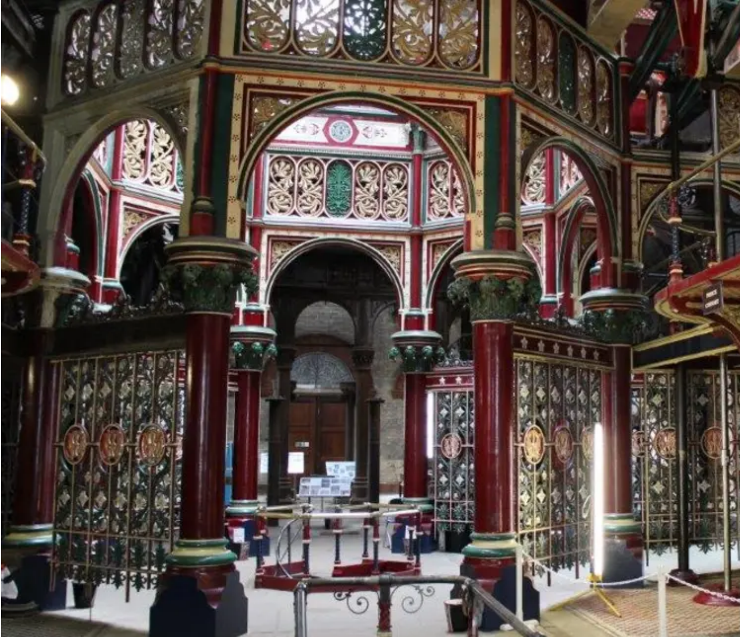
Ornate metalwork at Crossness Pumping Station
