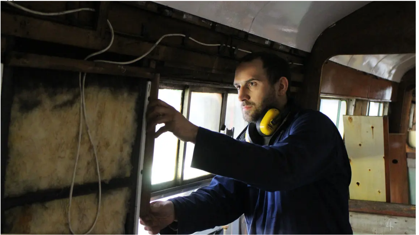
Apprentice Alastair Steele gets to work on a heritage train
