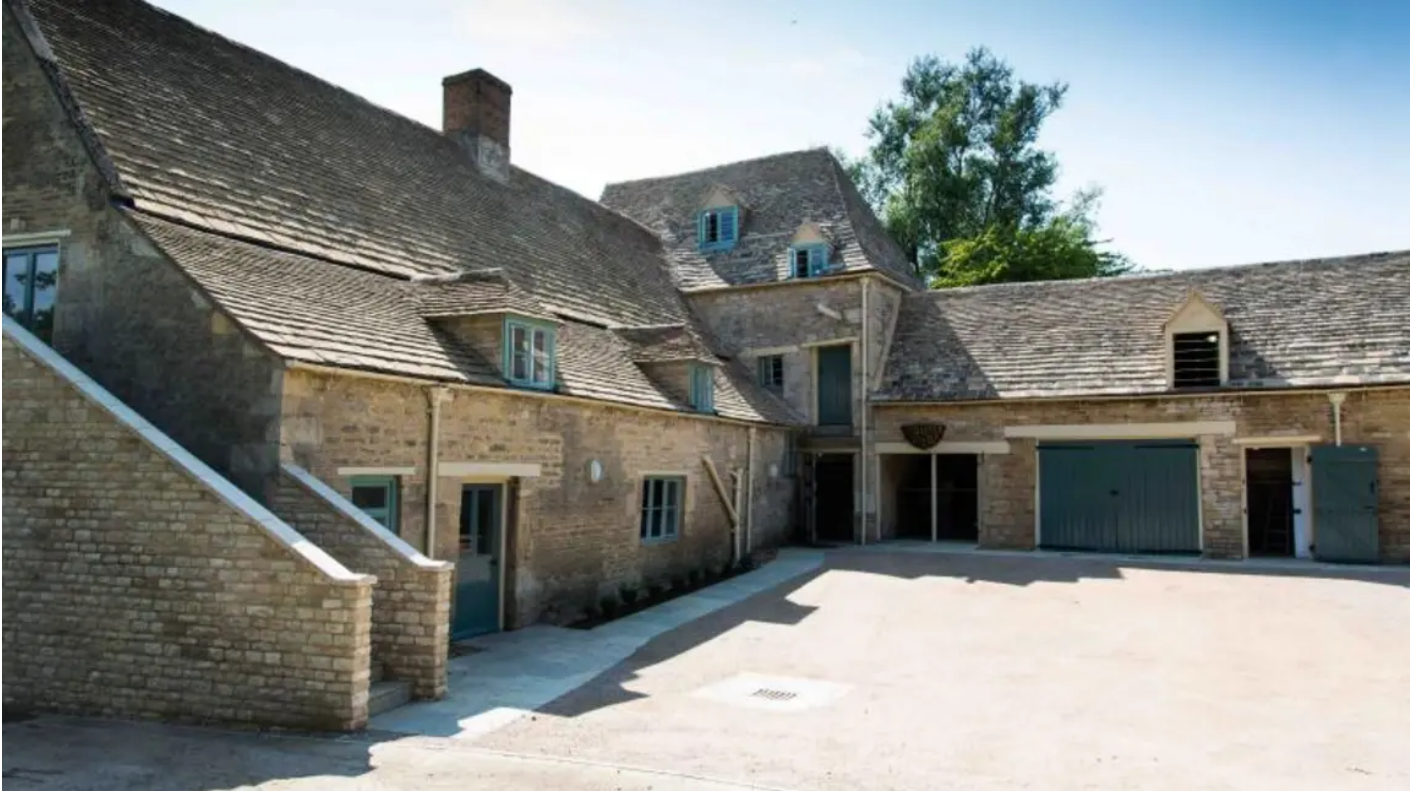
Sacrewell Mill after the restoration
