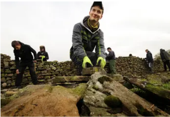
A trainee learns dry stone walling on an HLF project in the North West
