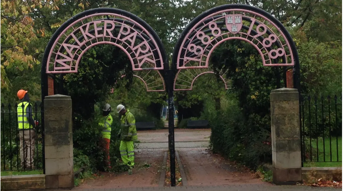
Scrub clearing by Walker Park entrance
