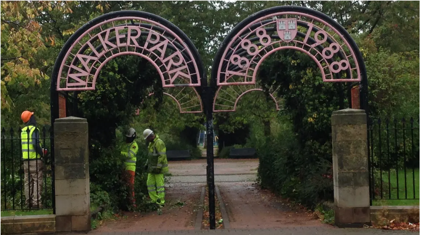
Scrub clearing by Walker Park entrance
