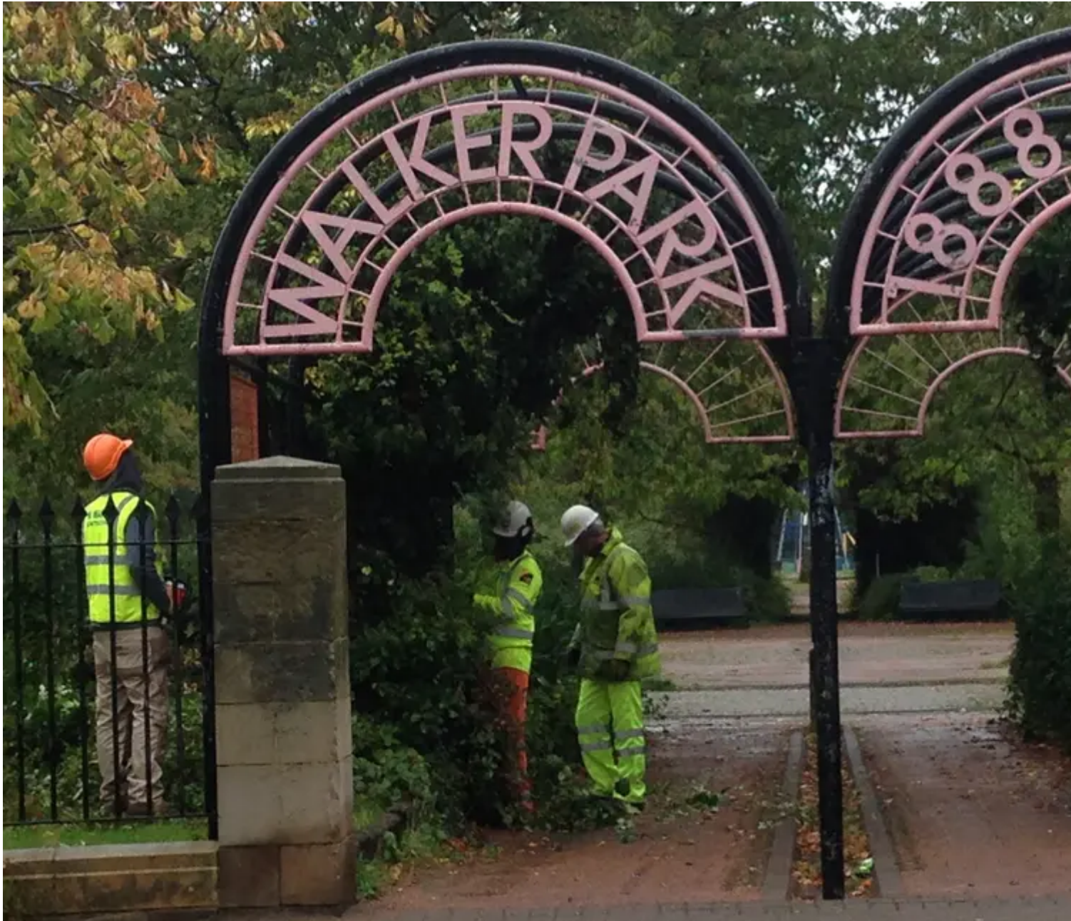
Scrub clearing by Walker Park entrance
