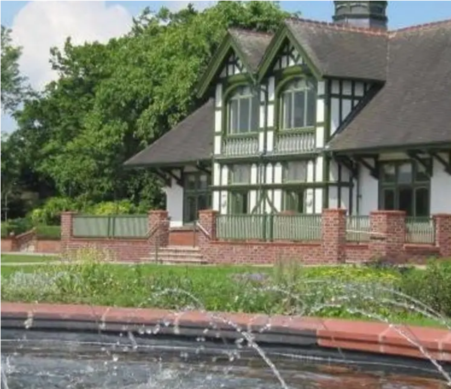
Pavilion at Burslem Park
