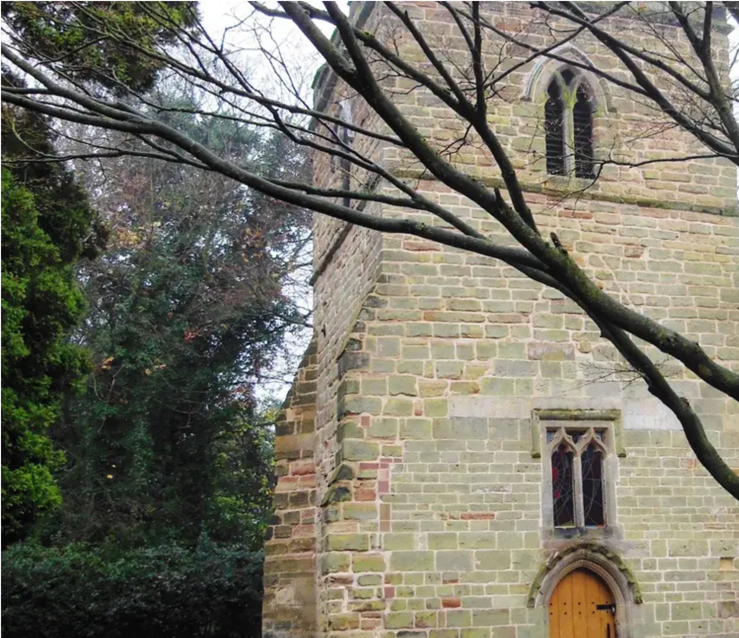
Bramcote Old Church Tower
