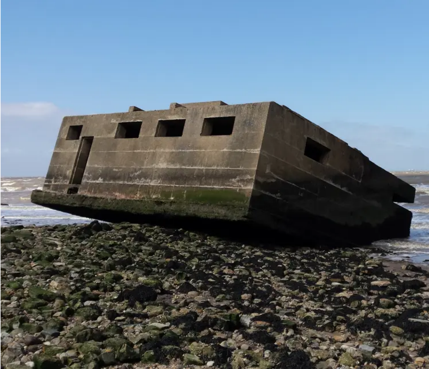
Pill box disappearing in to the sea on the Isle of Sheppey CITiZAN
