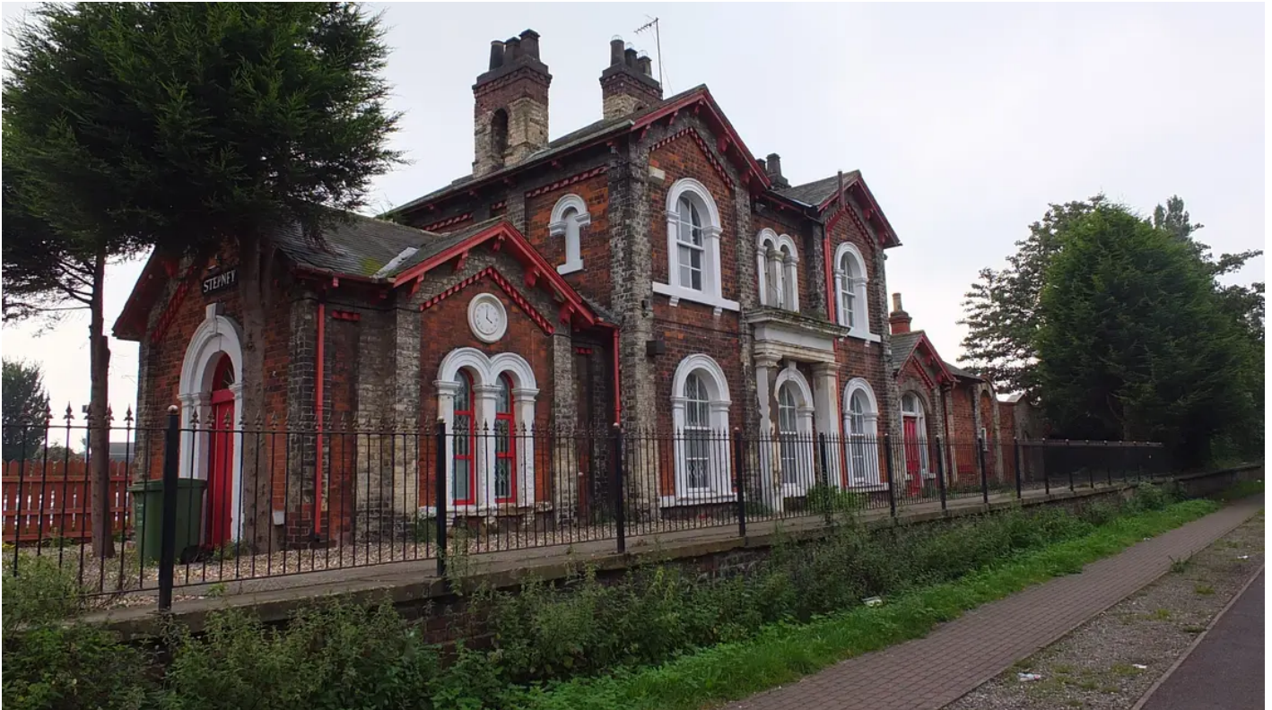
Stepney Station, a key part of the scheme
