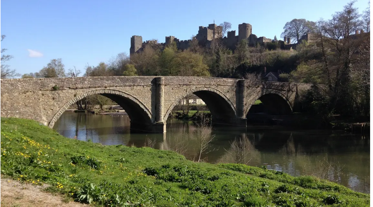
Dinham Bridge, Ludlow
