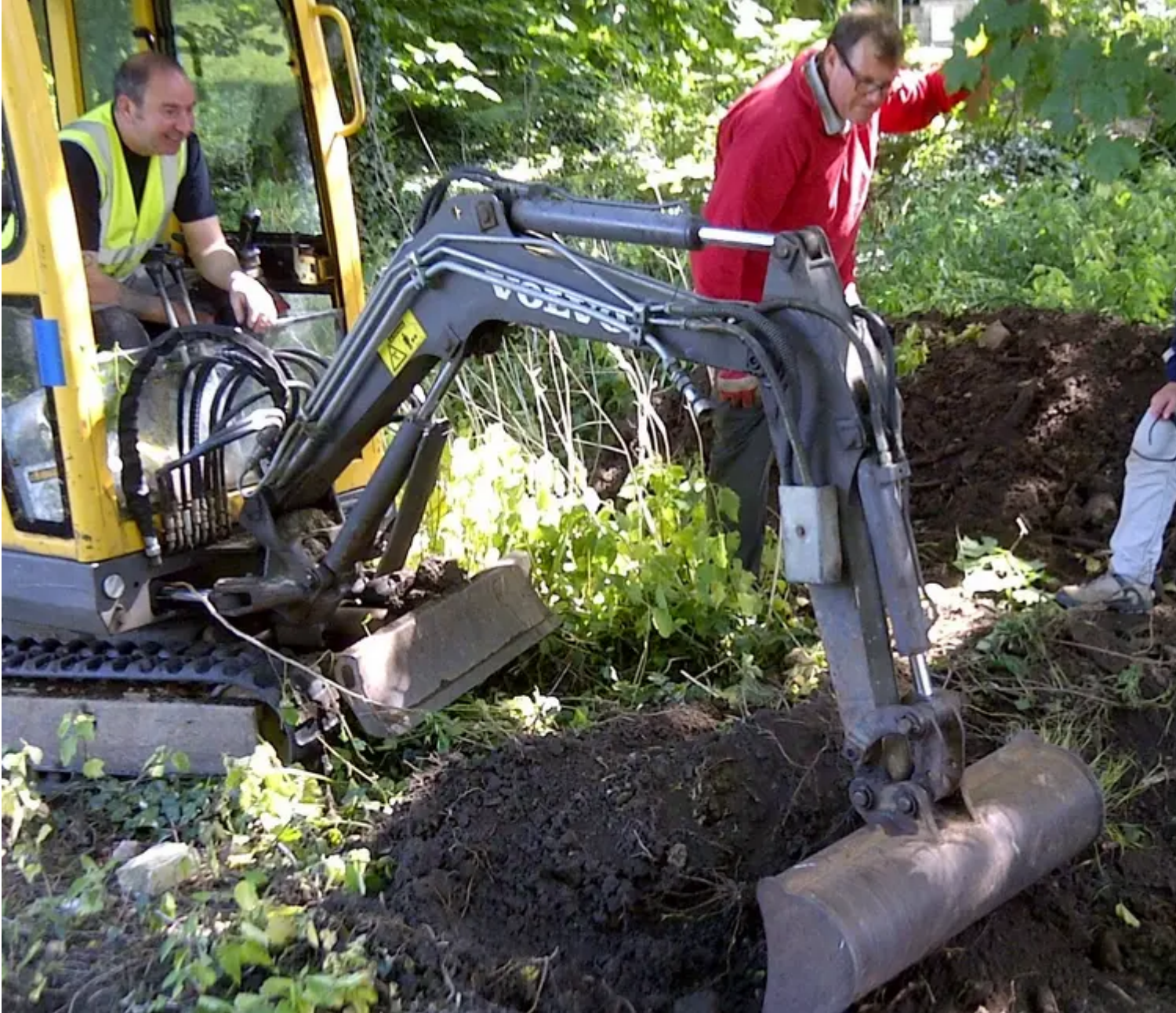
Volunteers extending and opening the first trench
