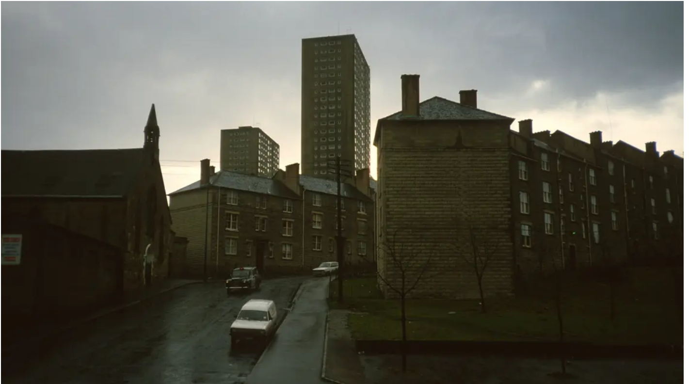
Royston B in Glasgow, shown in its partly-demolished state
