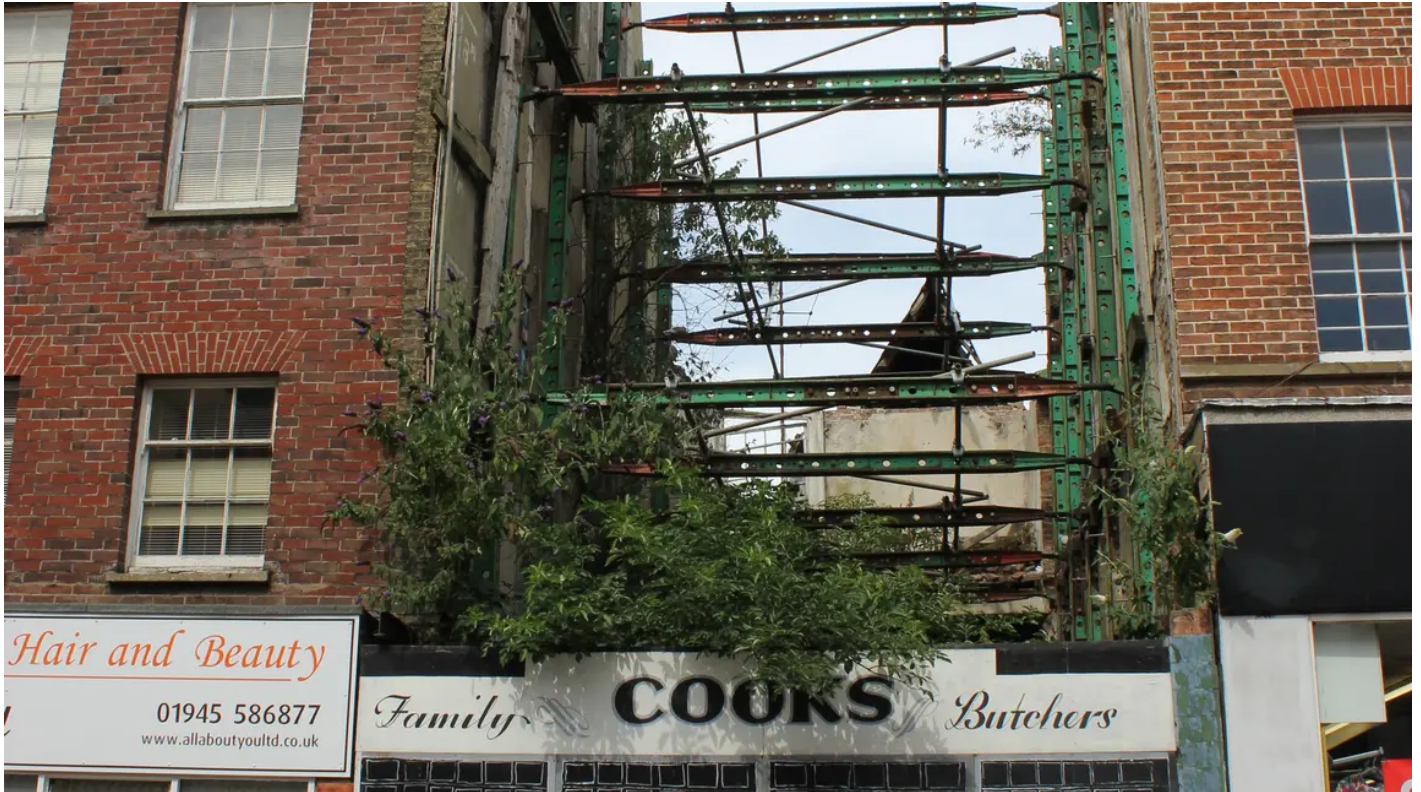
Wisbech High Street Project, Cambridgeshire, East of England
