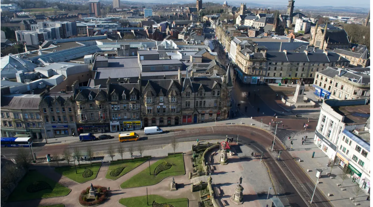
Aerial view of Paisley town centre
