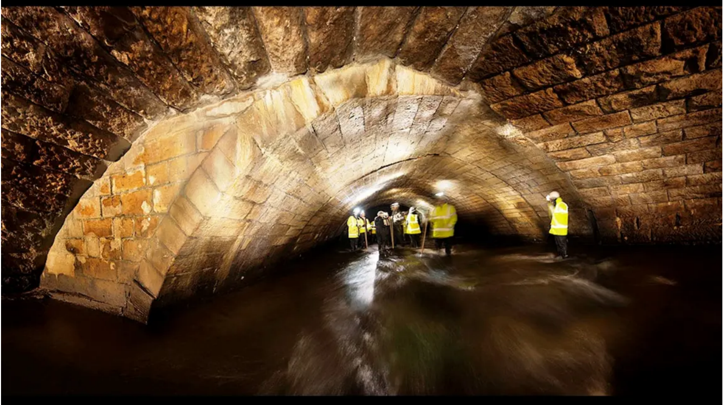
People inspecting the River Roch's medieval bridge Andrew Brookes
