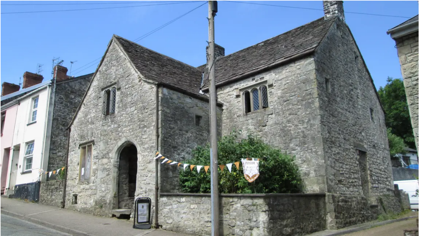
St John's House, Bridgend
