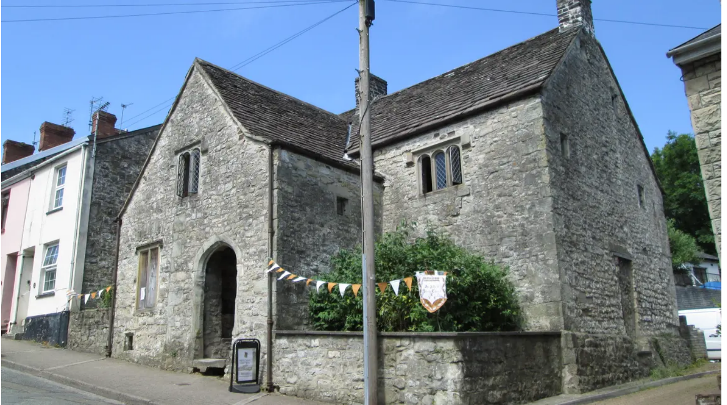
St John's House, Bridgend
