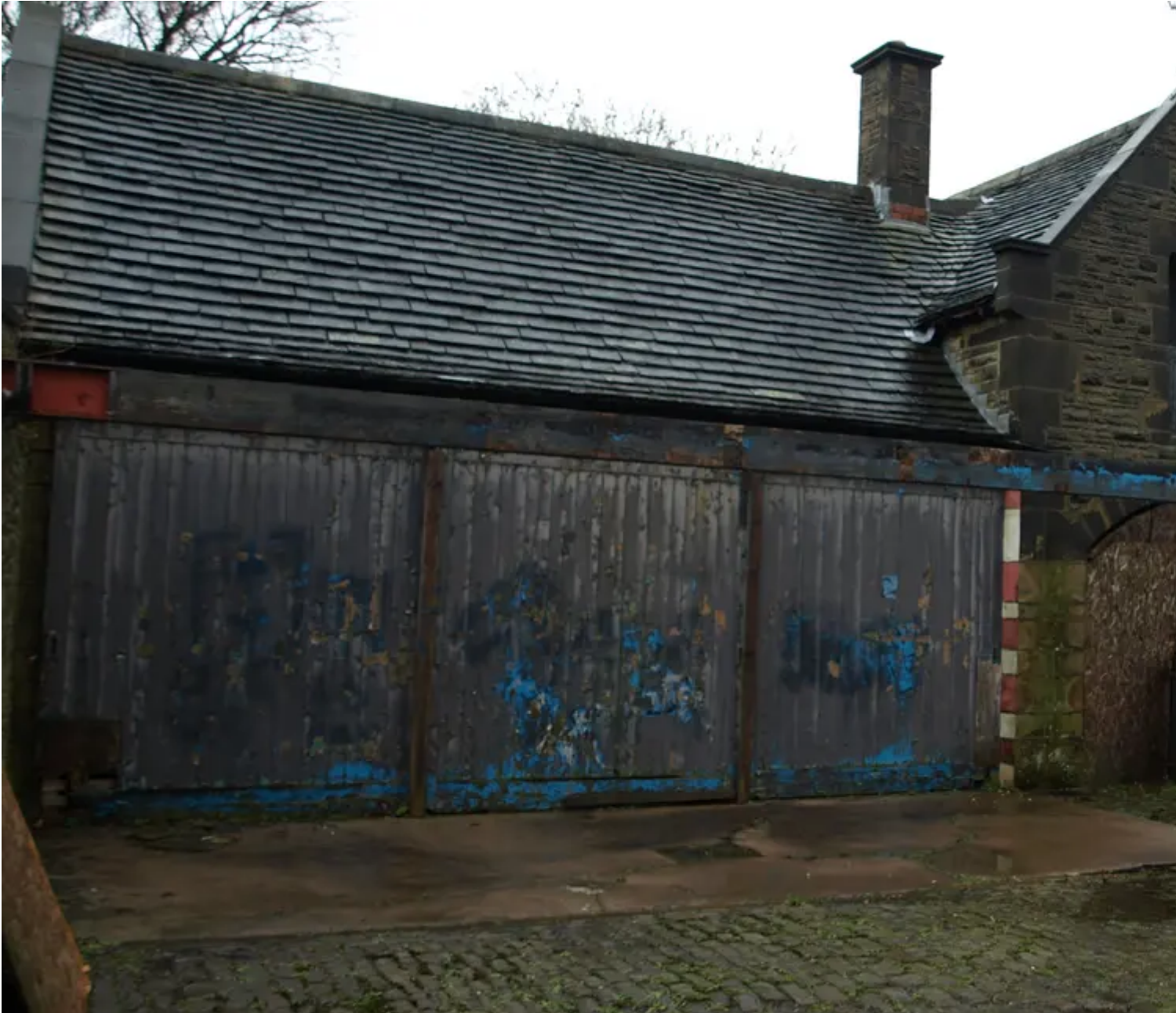
Stables and Motor House at Haworth Art Gallery
