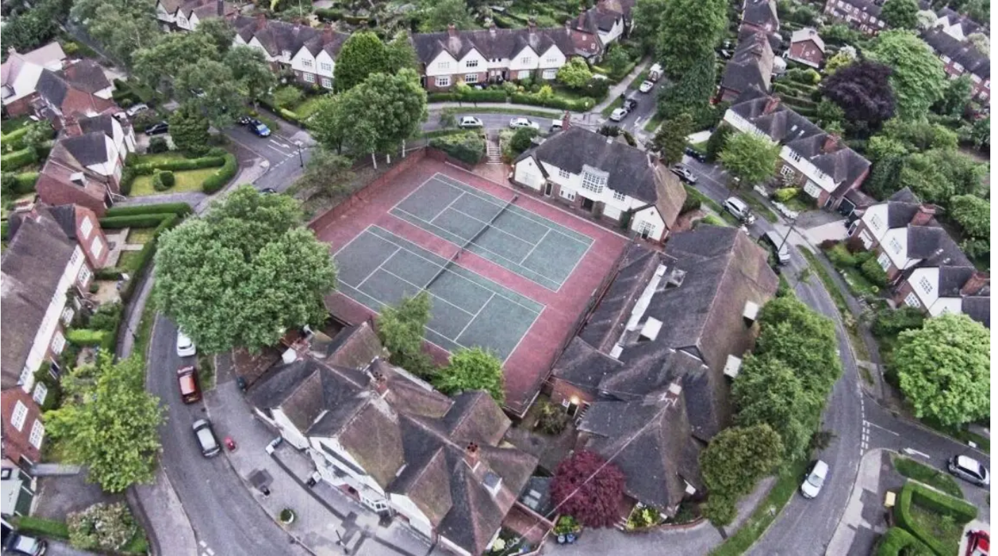
Aerial shot of Moor Pool community hall
