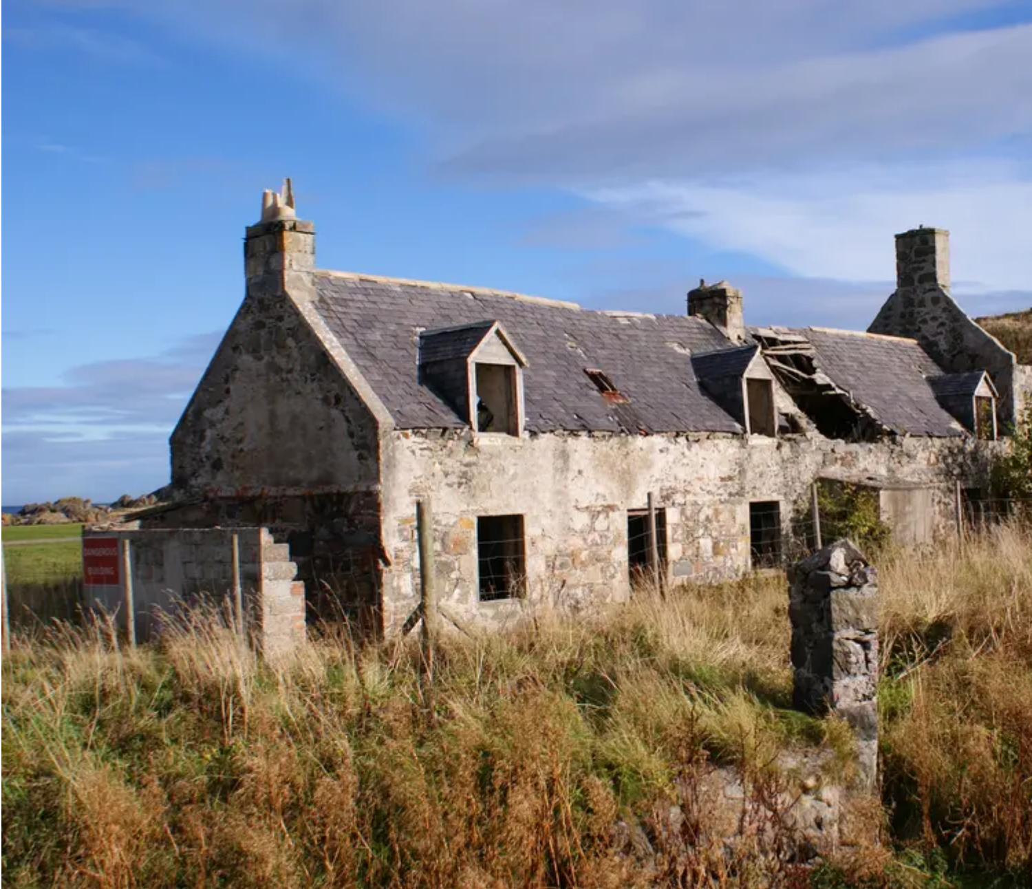
Exterior view of Portsoy Bunkhouse
