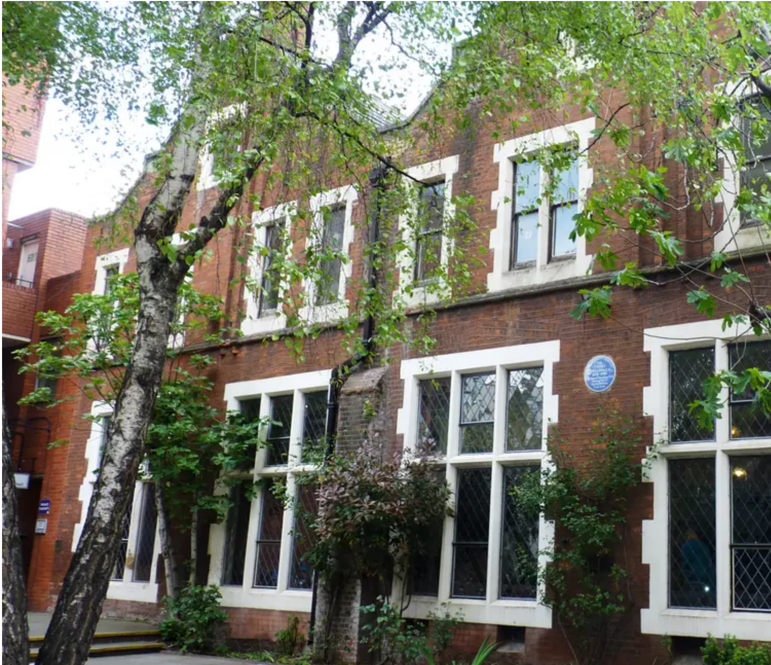
Exterior of Toynee Hall
