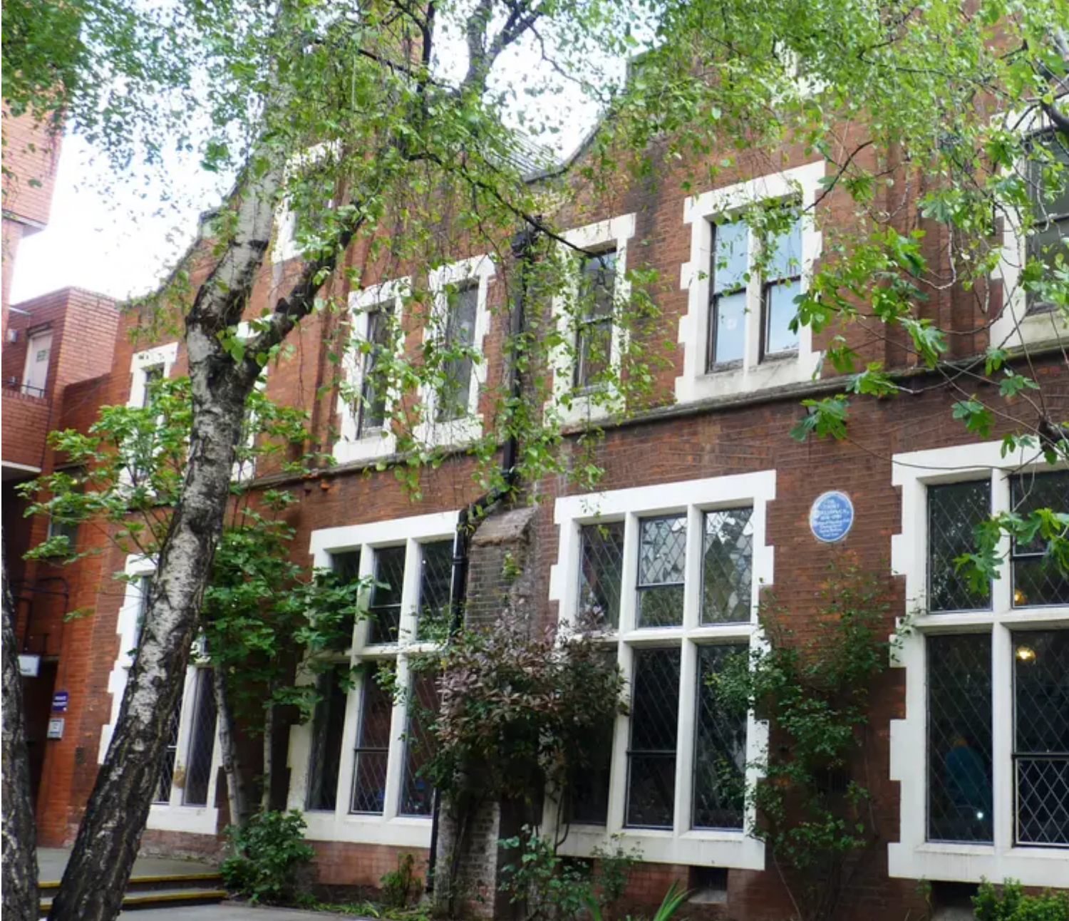
Exterior of Toynee Hall
