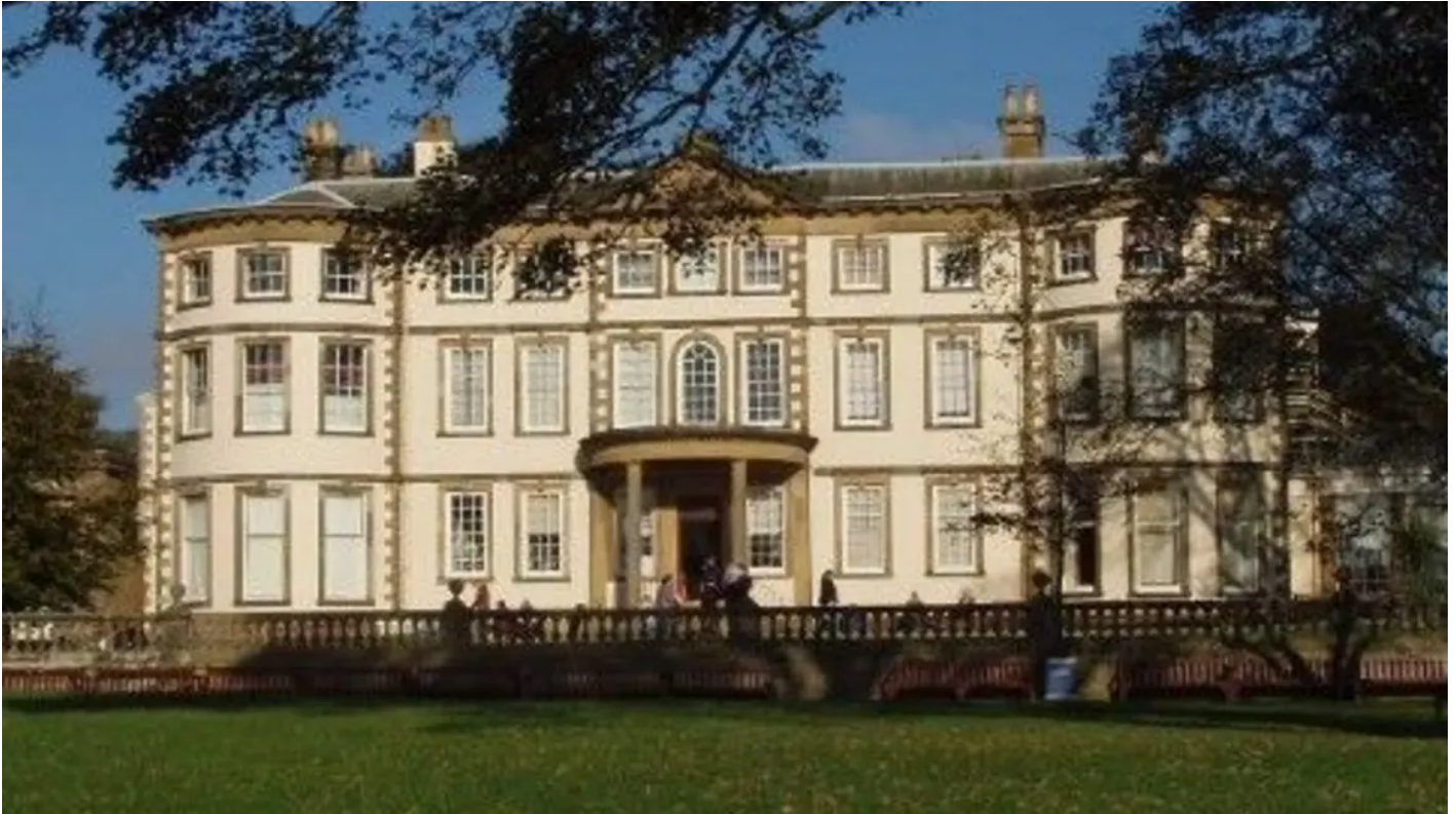
Sewerby Hall reopens after restoration
