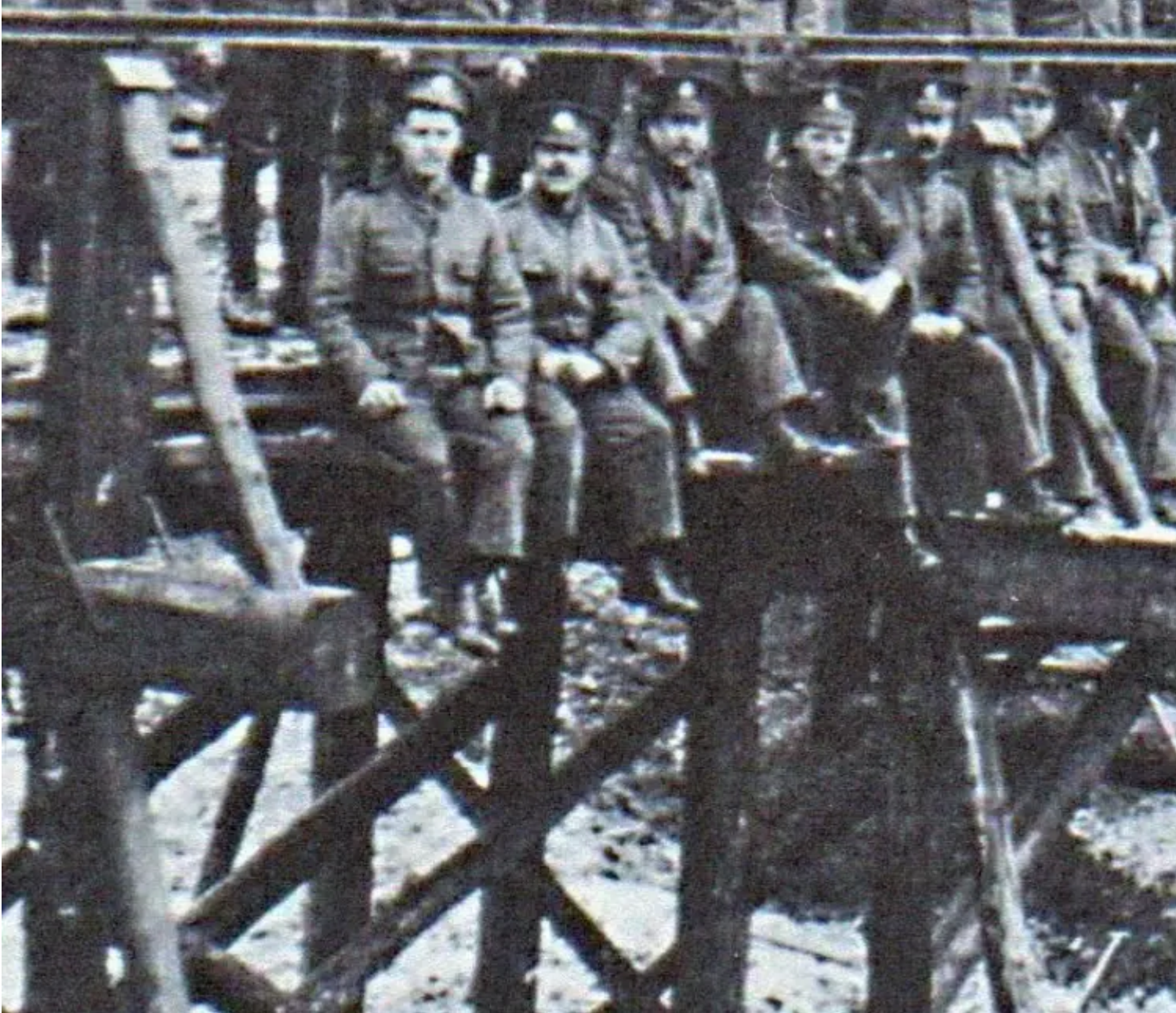
Bridging training over the Marlow Common clay quarry
