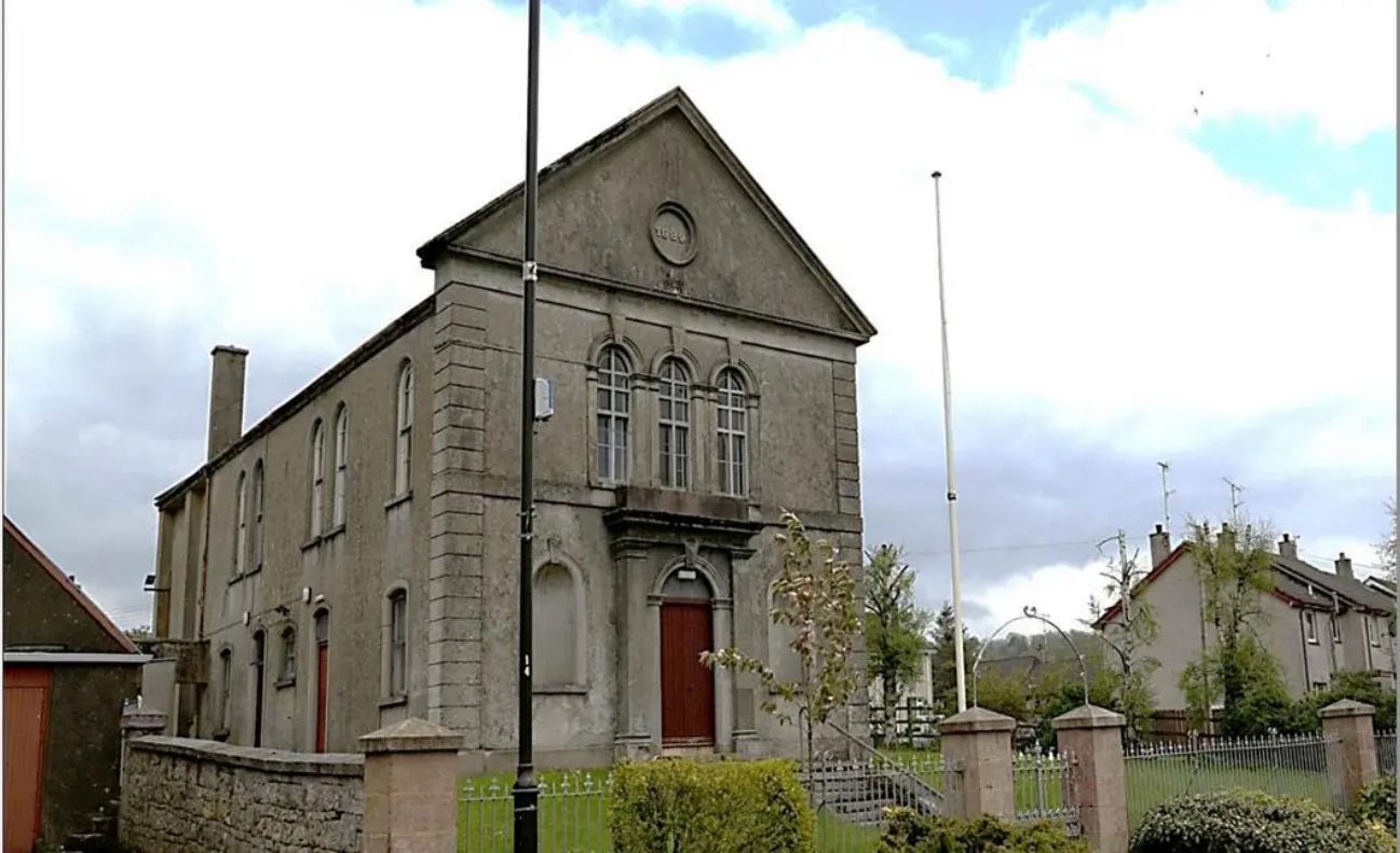
View of the outside of Derrygonnelly Orange Hall building
