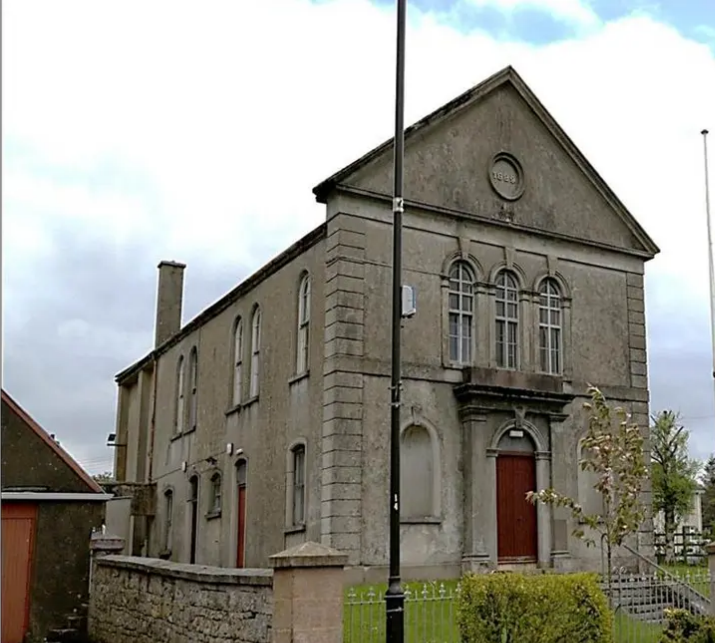
View of the outside of Derrygonnelly Orange Hall building
