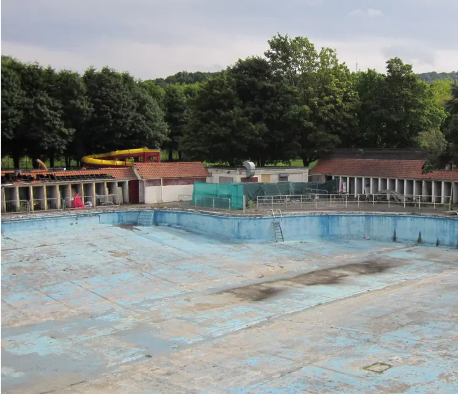
Current condition of Ynysangharad Park Lido
