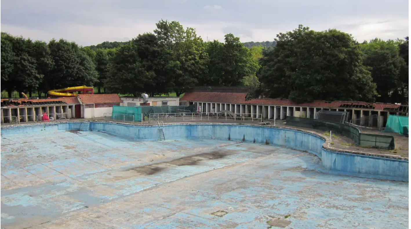
Current condition of Ynysangharad Park Lido
