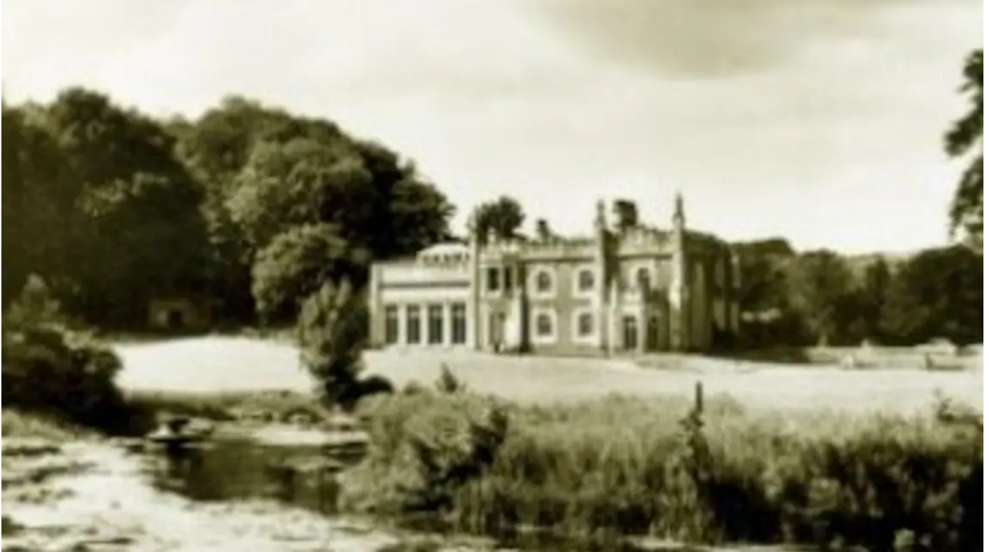
Archive image of the Gothic revival Manor House at Kearsney Abbey
