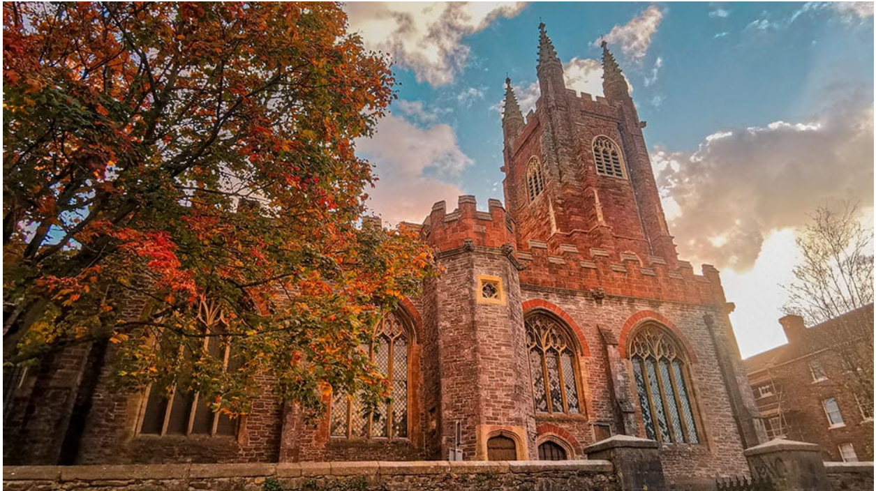
St Mary's Church in Totnes will power their new heating system using renewable energy. Photo: St Mary's Totnes.
