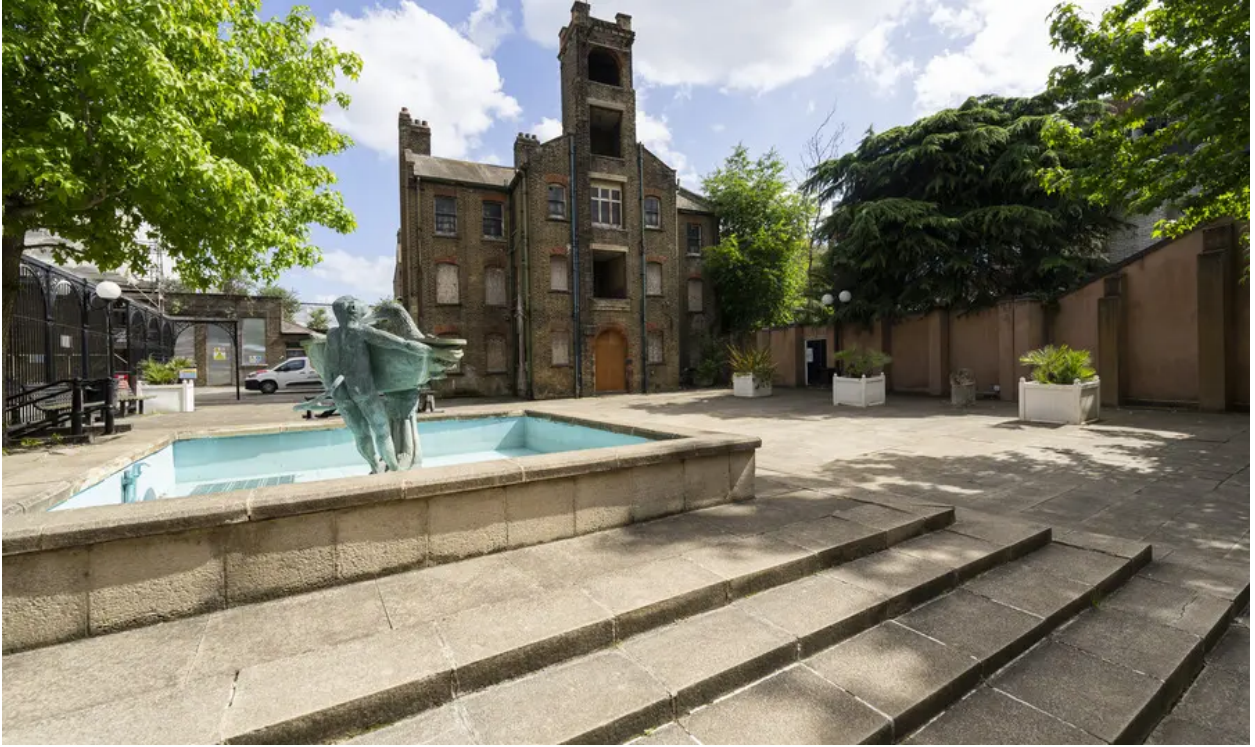
Alice Billings House before work started for its transformational project. Credit: Andrew Baker Photographer.
