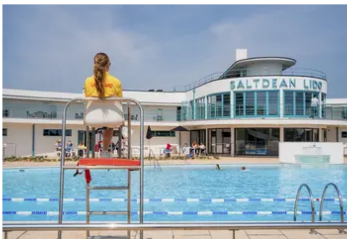
The restored Saltdean Lido. Credit: Xavier Buendia.
