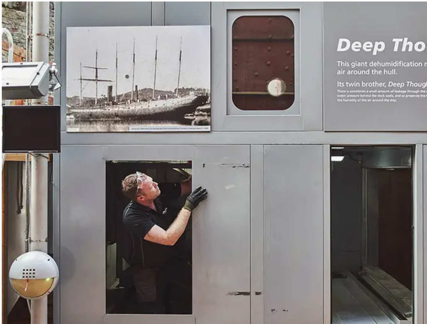
Refitting the dehumidifier fans that preserve SS Great Britain. Photo: Adam Gasson / Munters / SS Great Britain Trust.
