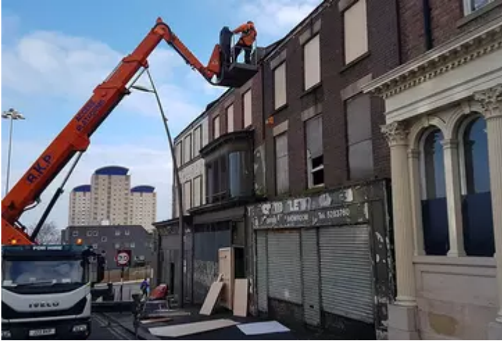
Georgian houses in Sunderland before restoration
