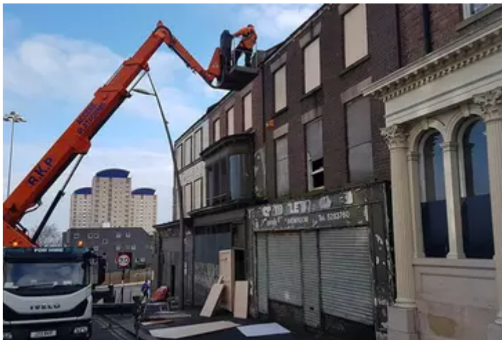
Georgian houses in Sunderland before restoration
