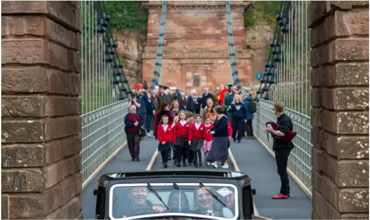
A vintage car and school children cross the Union Chain Bridge as it reopens to traffic. Credit: Northumberland County Council
