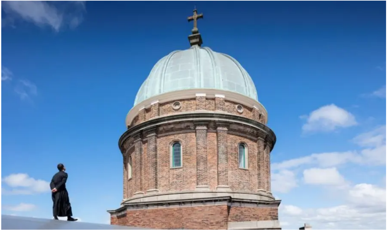
The newly conserved dome of the Church of Saints Peter and Paul and Saint Philomena. Credit: Historic England Archive
