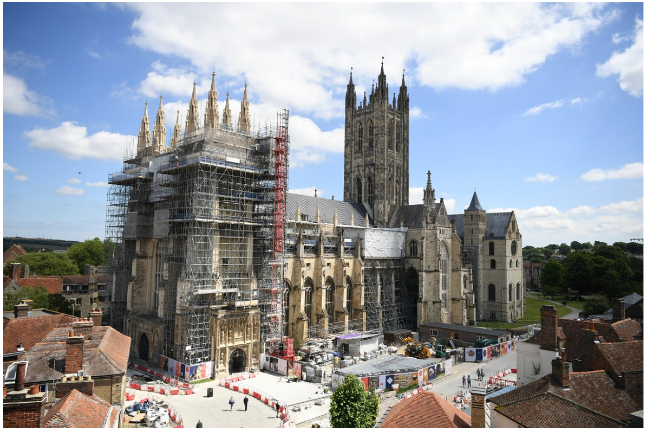
Canterbury Cathedral undergoing restoration
