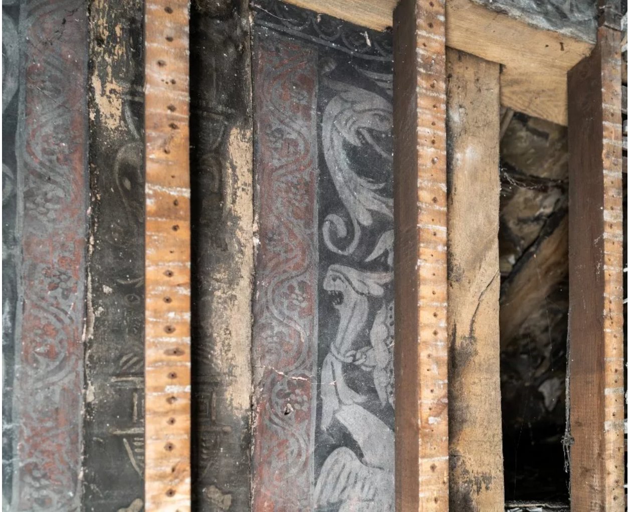
Close up of roaring griffins shown in the Tudor wall paintings discovered at Calverley Old Hall. Credit: The Landmark Trust
