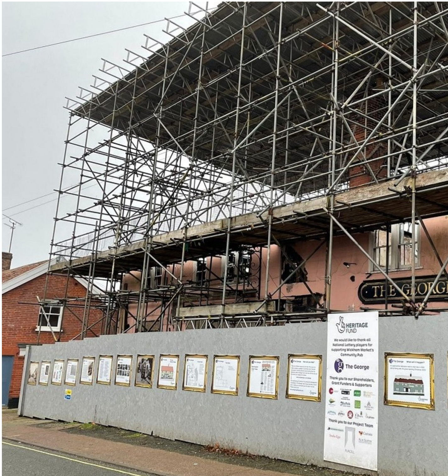
Scaffolding outside the pub to prepare for construction. Credit: Bill Wolff-Evans
