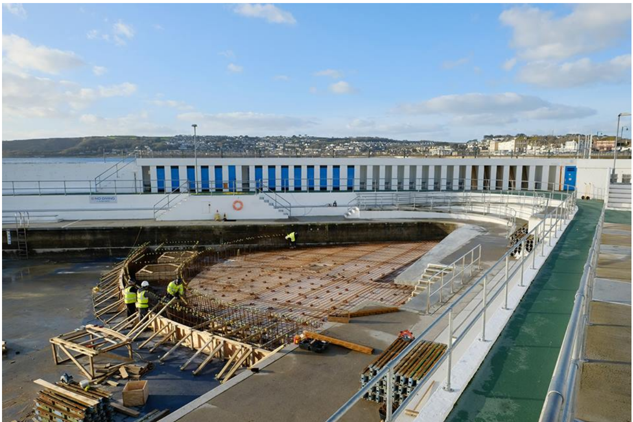
Jubilee pool under construction
