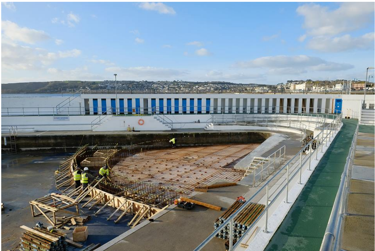
Jubilee pool under construction
