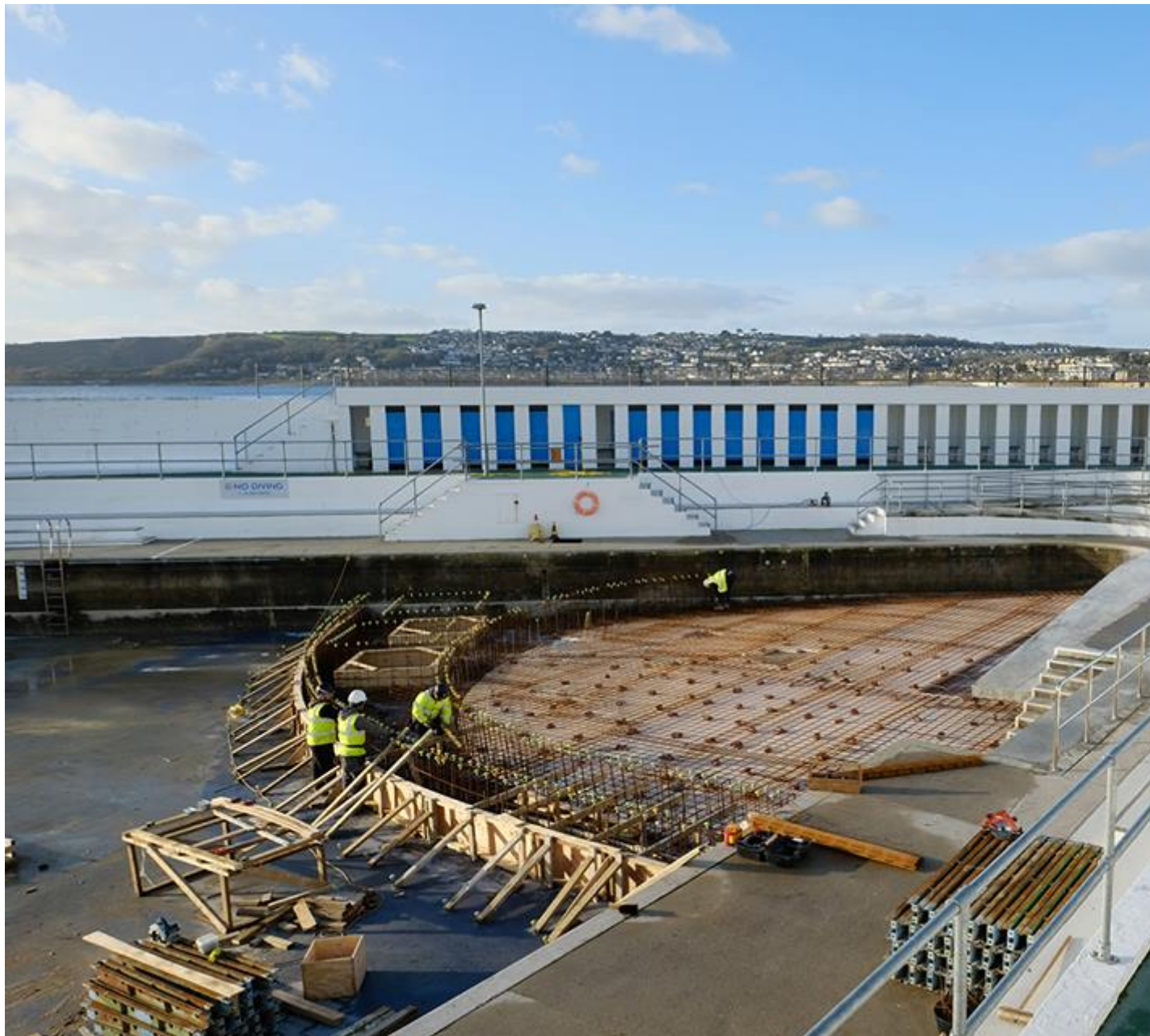
Jubilee pool under construction
