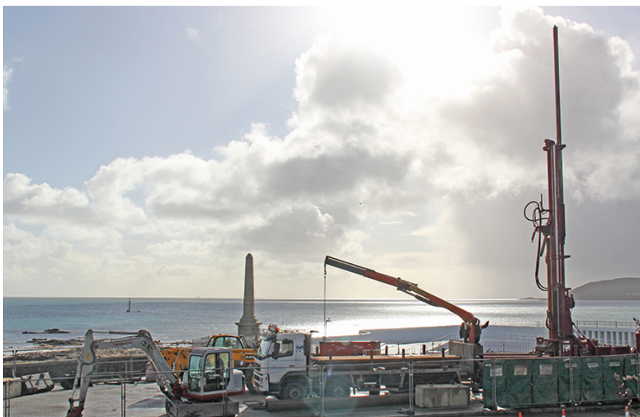
Construction of the geothermal well at Jubilee Pool
