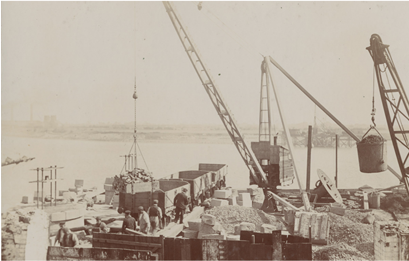
Workers building the bridge, which originally opened in 1906.
