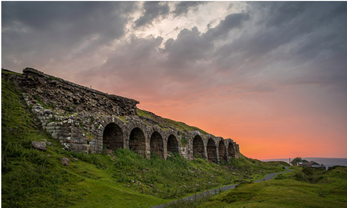
Rosedale Bank Top, North Yorkshire. Credit: Paddy Chambers
