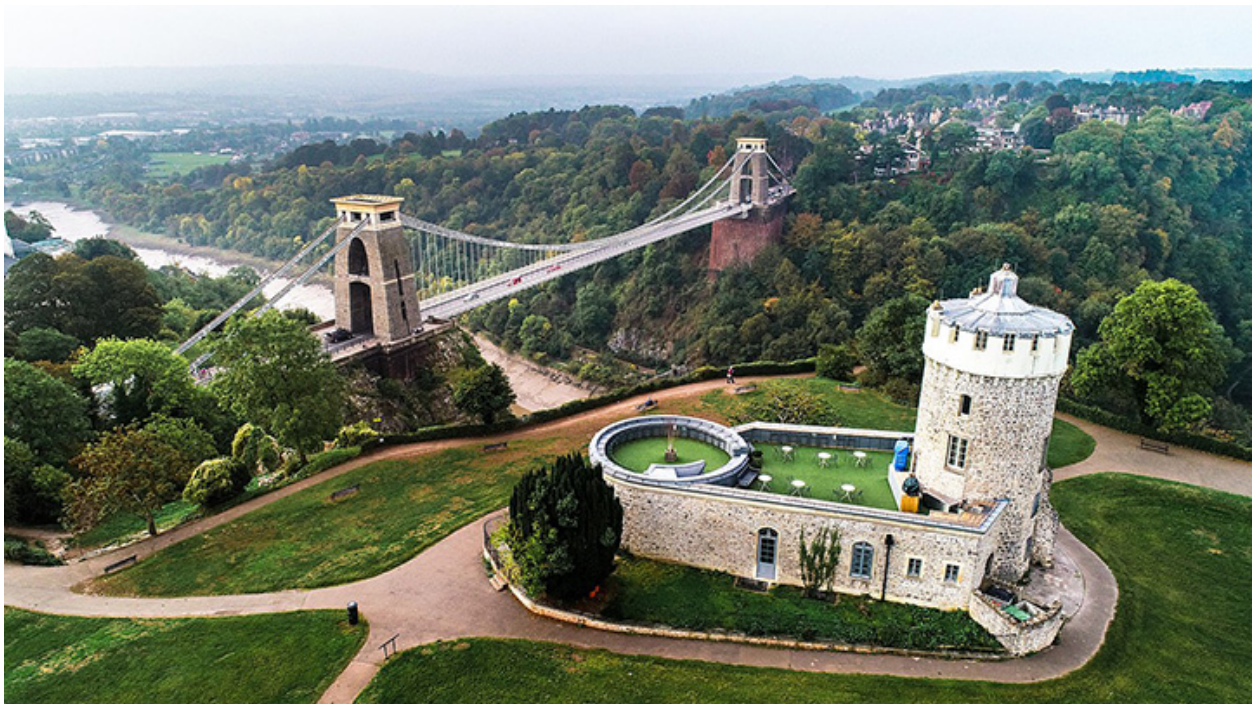
Clifton Suspension Bridge and the Observatory in Bristol, England. Credit: Chris Lathom-Sharp, Wikimedia Commons, CC BY-SA 4.0
