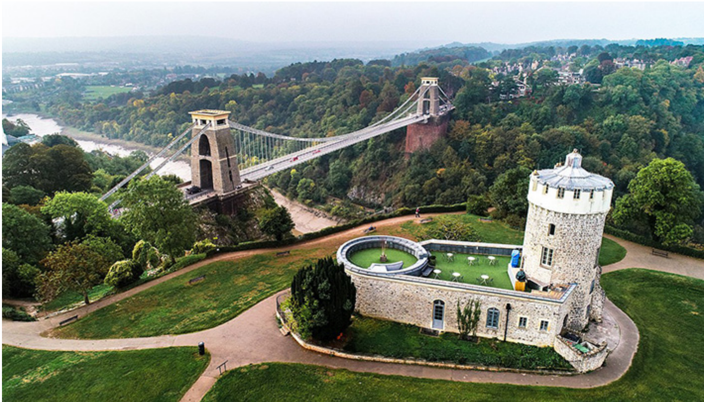
Clifton Suspension Bridge and the Observatory in Bristol, England. Credit: Chris Lathom-Sharp, Wikimedia Commons, CC BY-SA 4.0
