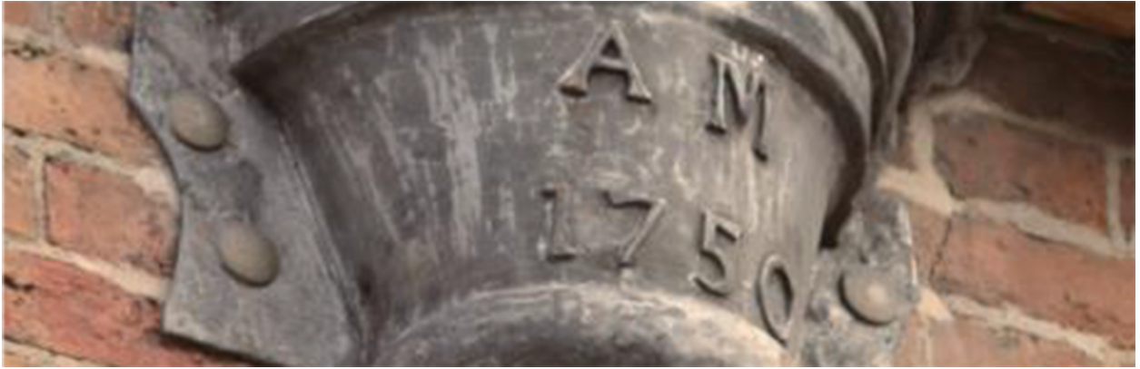
The drainpipe hopper with Ann's initials. Credit: Nottingham City Council
