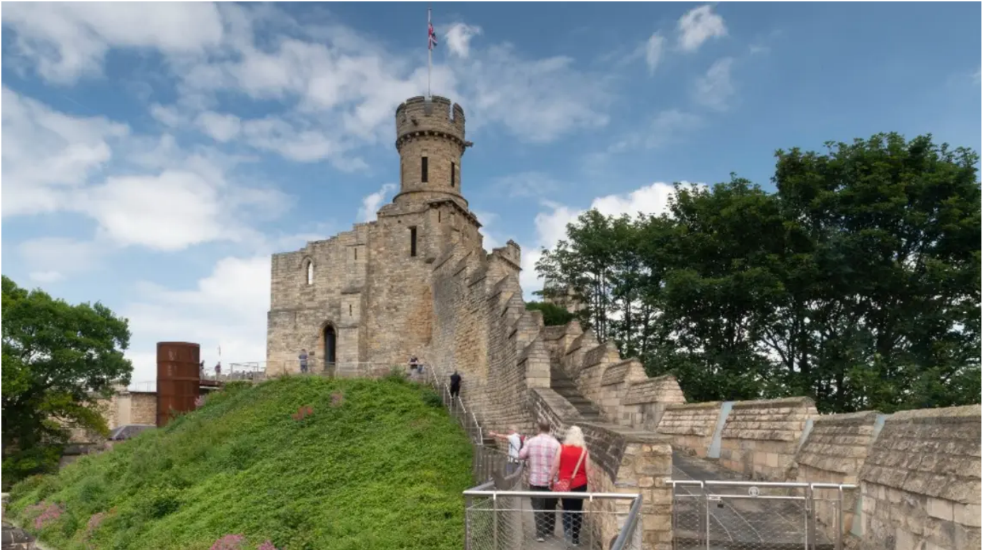
Lincoln Castle. Credit: Colin McLean Photography Safeguarding our historic buildings, monuments and archaeology for future generations.
