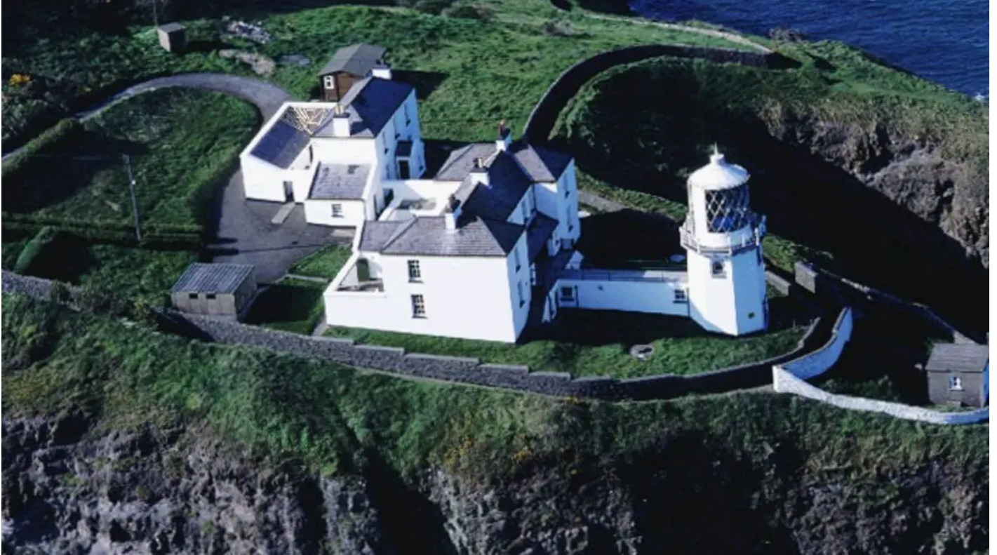
Lighthouse heritage to benefit from EYCH18 funding
