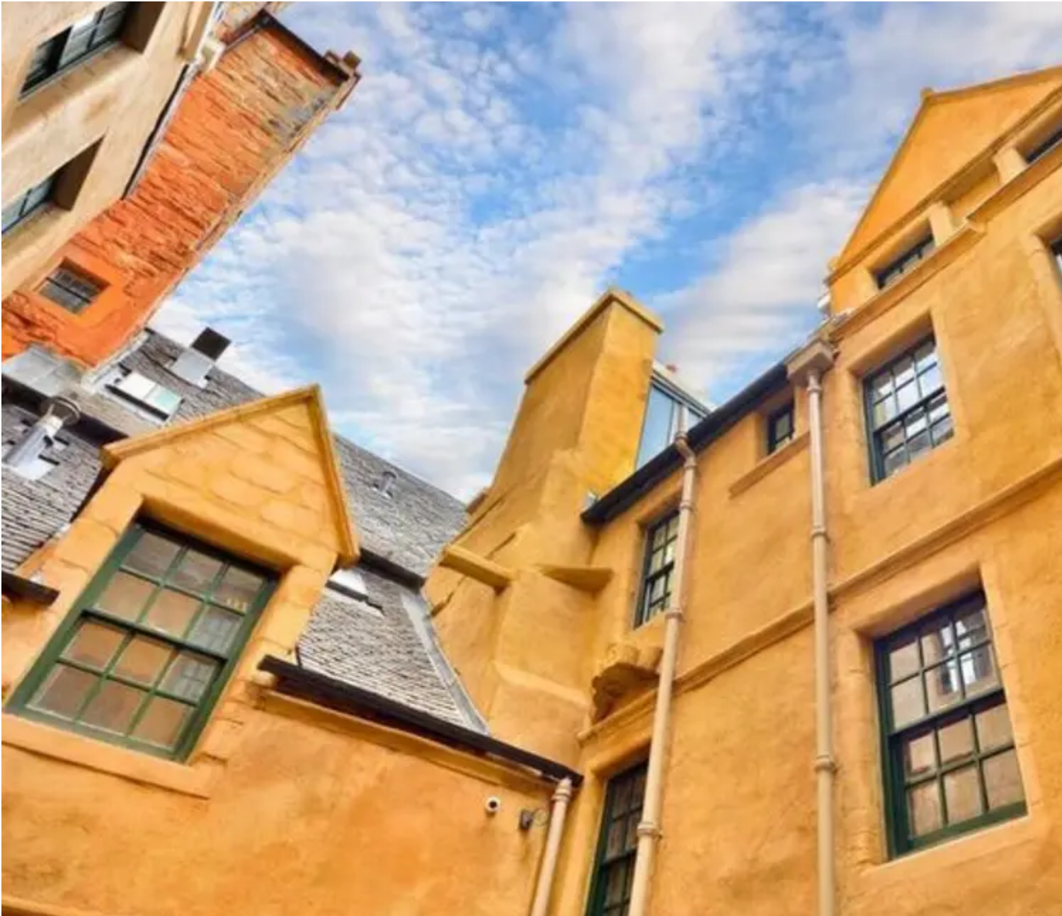
Restored Patrick Geddes Centre for Learning and Conservation
