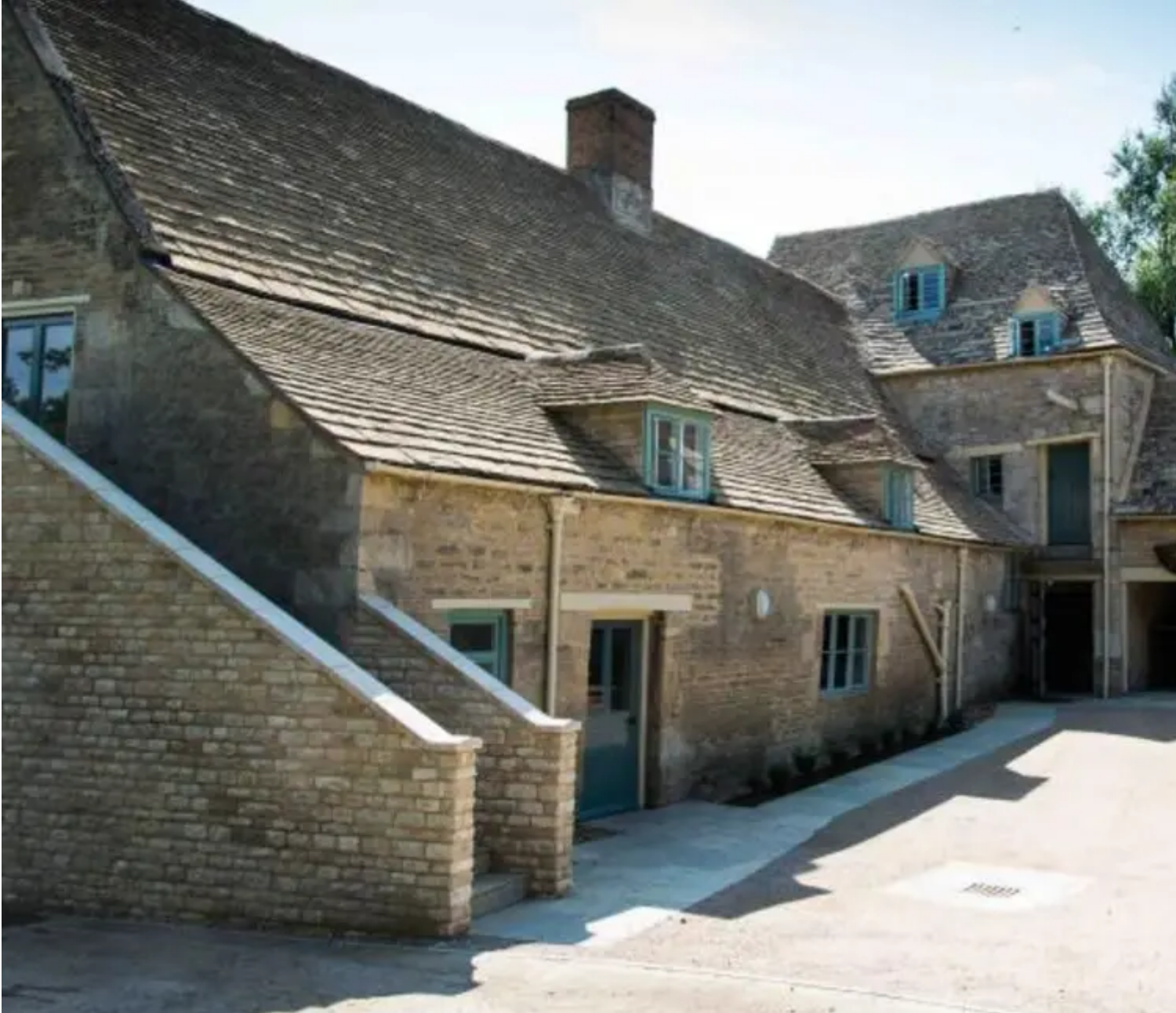
Sacrewell Mill after the restoration
