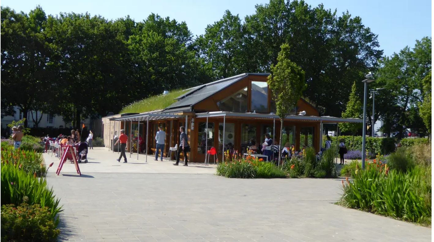
The Level, Brighton after its National Lottery-funded restoration
