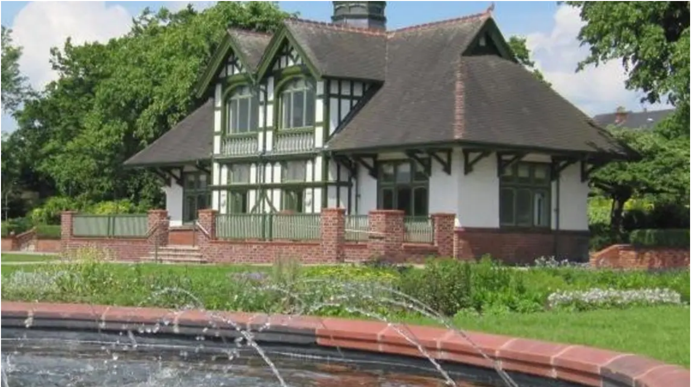
Pavilion at Burslem Park
