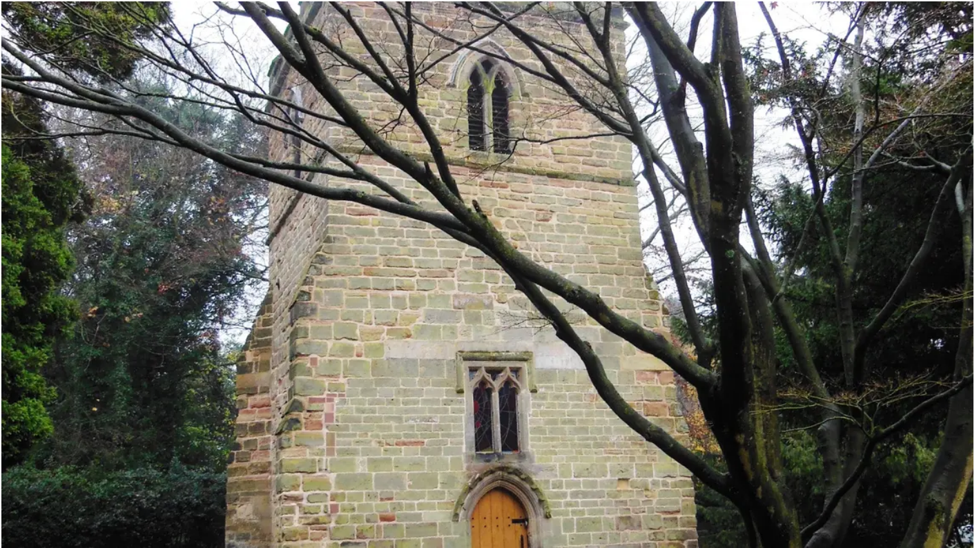
Bramcote Old Church Tower
