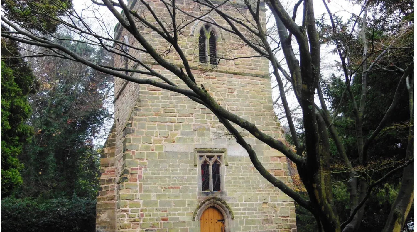
Bramcote Old Church Tower
