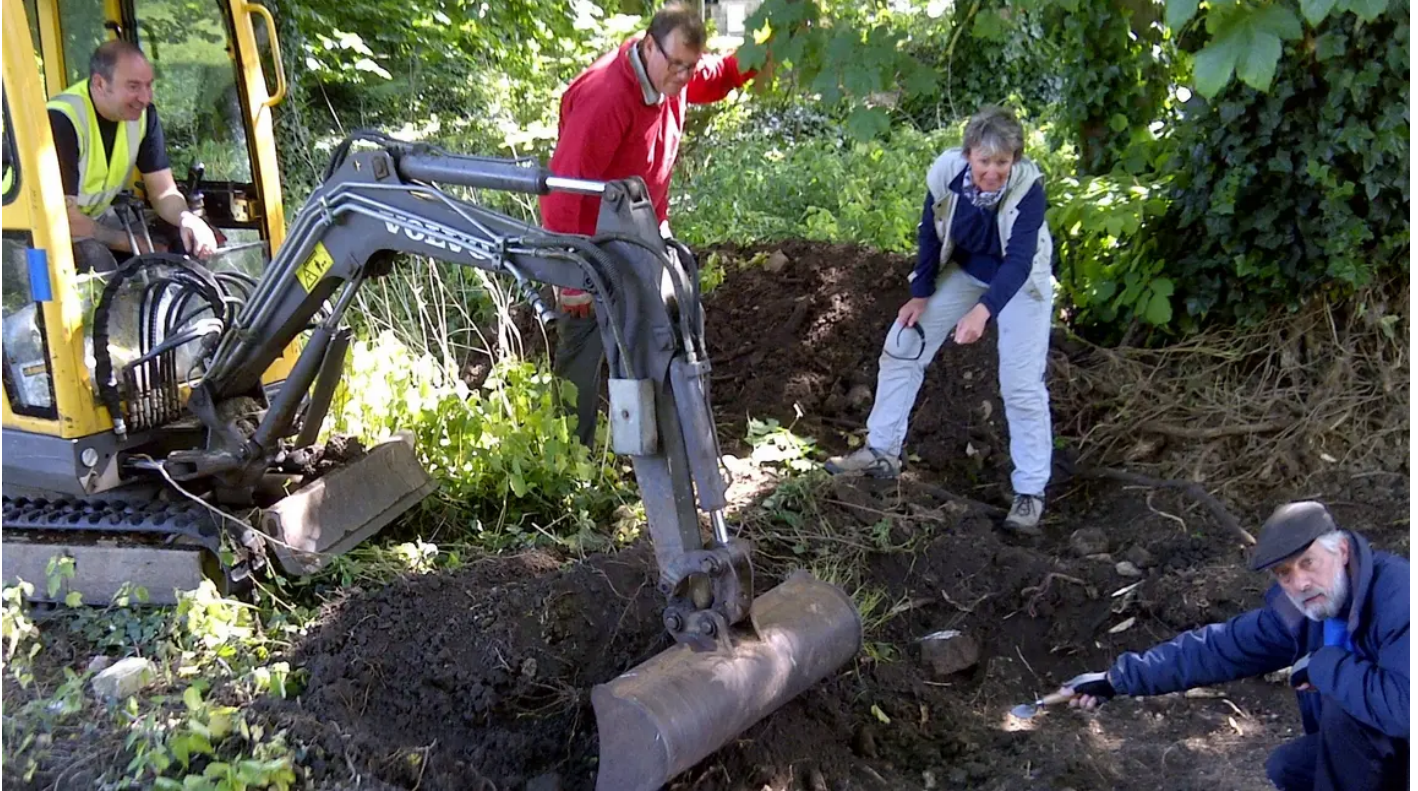
Volunteers extending and opening the first trench
