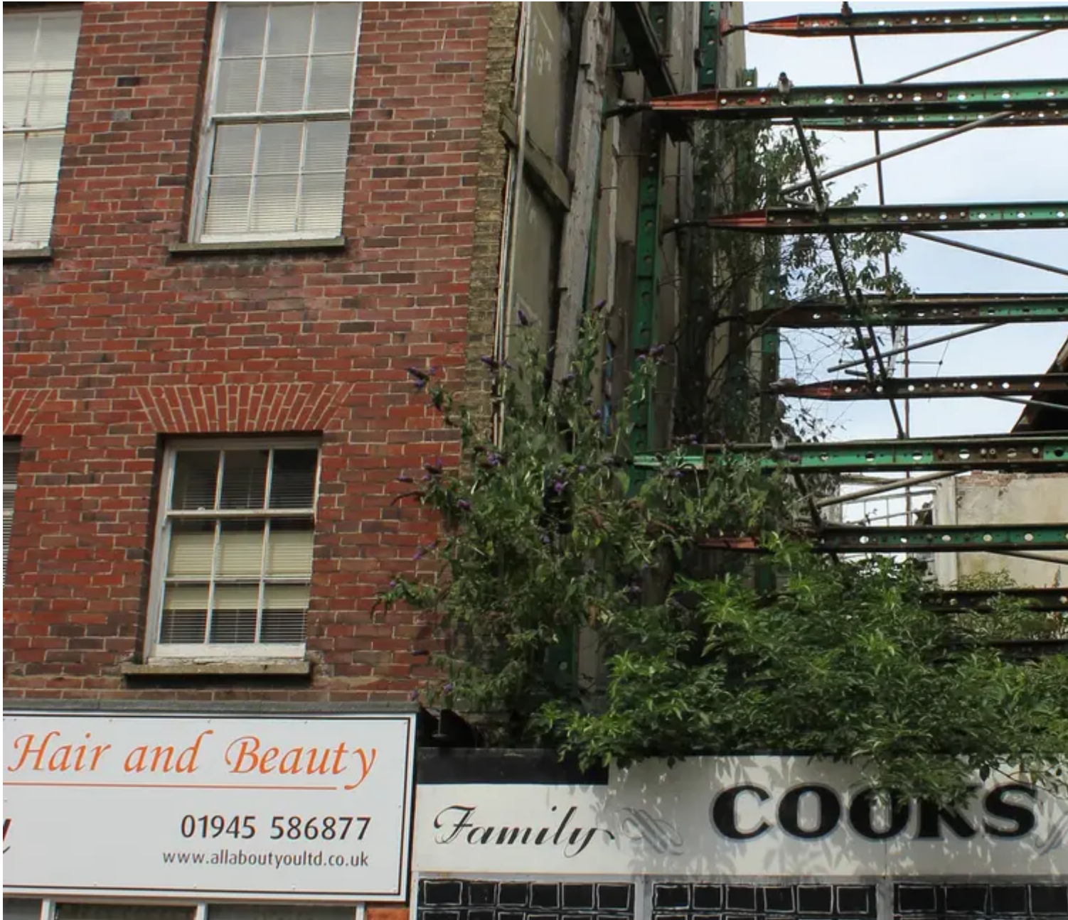
Wisbech High Street Project, Cambridgeshire, East of England
